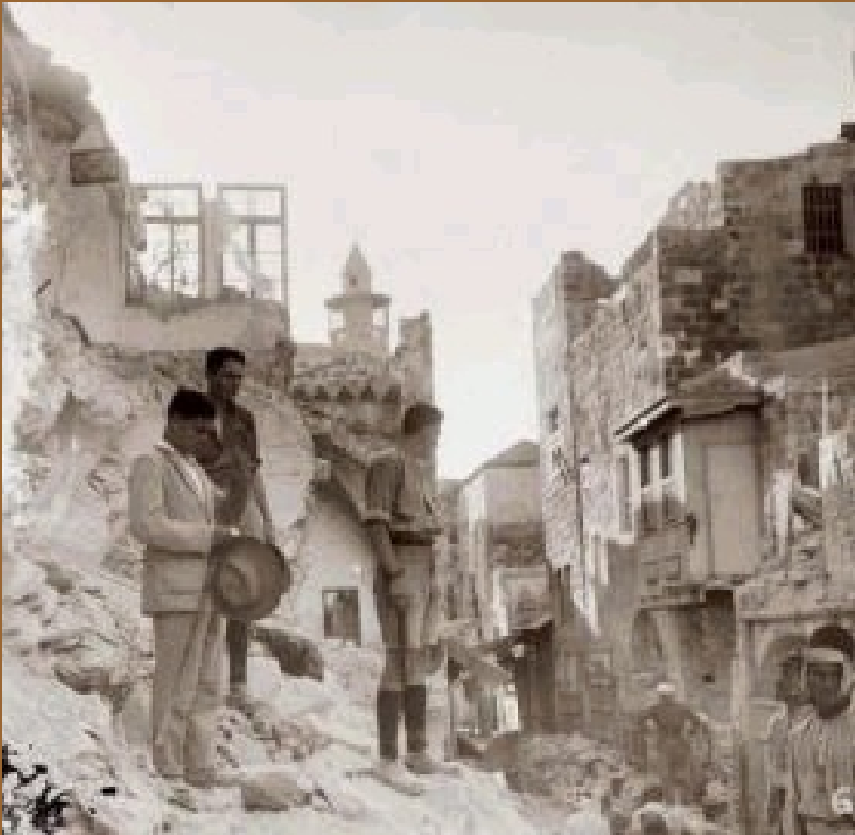
1927 Jerusalem 6.3 Earthquake Rev. 11:13 earthquake will be similar.
